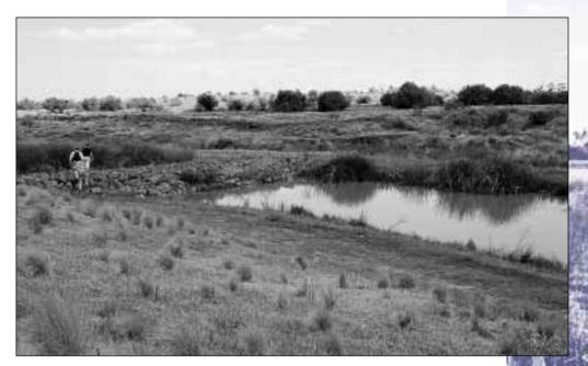
Constructed wetland inlet zone with a porous rock embankment to distribute flows evenly across the macrophyte zone. The by-pass weir is located on the far side of the open water area
