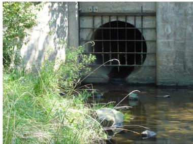
From here, the rain water may enter into storm catch basins or roadside ditches before eventually entering into a local freshwater brook, river, lake or into the ocean.
